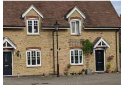
Yellow brick & decorative brick work above windows
