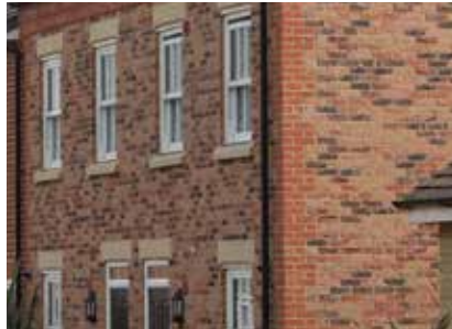
Combination of coloured bricks
